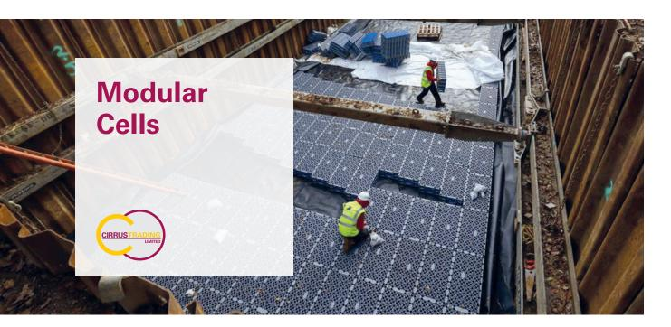
**Interlocking Modular Cells**, create strong, flexible, water attenuation or soakaway systems of any size, shape and depth to suit every ground and climatic condition.
